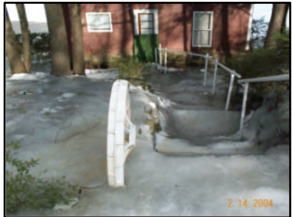
Ice buildup on the road has been spreading and encroaching on the camp of Eben & Jean Ellis.
