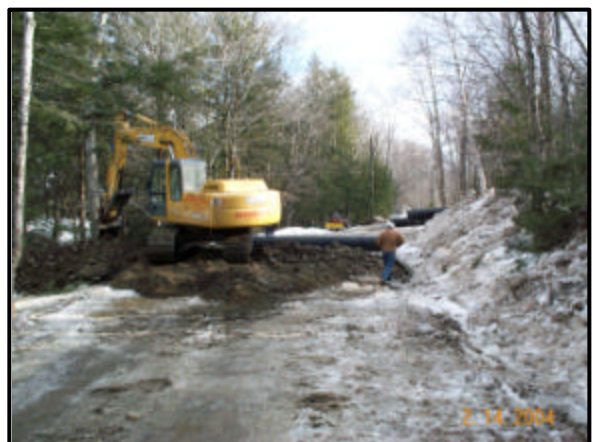
Many cubic yards of ice were removed and piled near the road before culvert installation.
